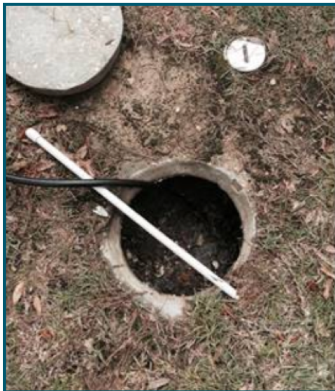
Figure 2. Home waste tank requiring pump out due to aerator not working for several years
